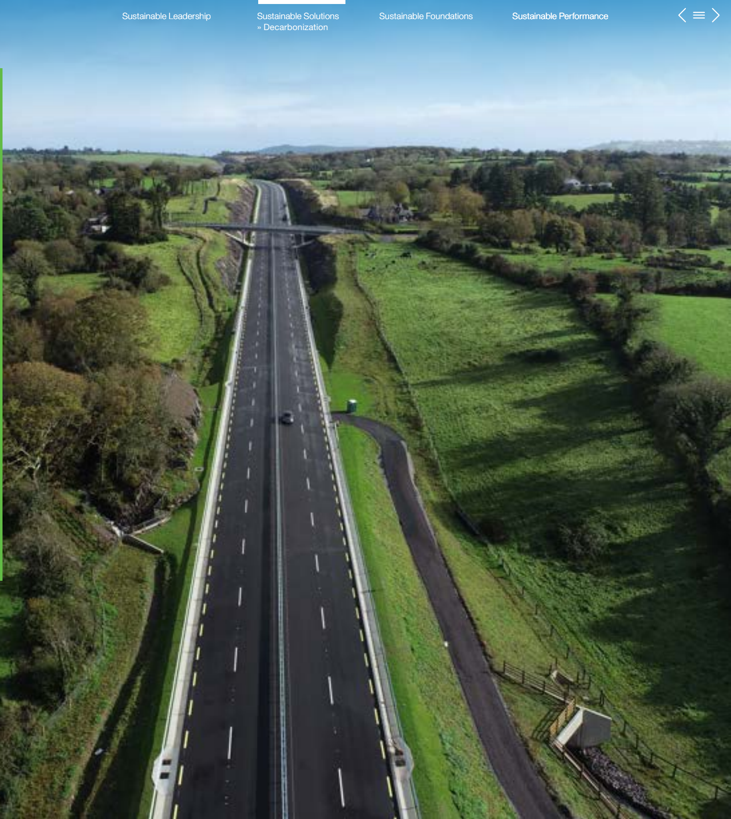
Lower-Carbon Asphalt using Recycled Materials on the N22 Dual Carriageway, Ireland Roadstone, CRH Europe Division
